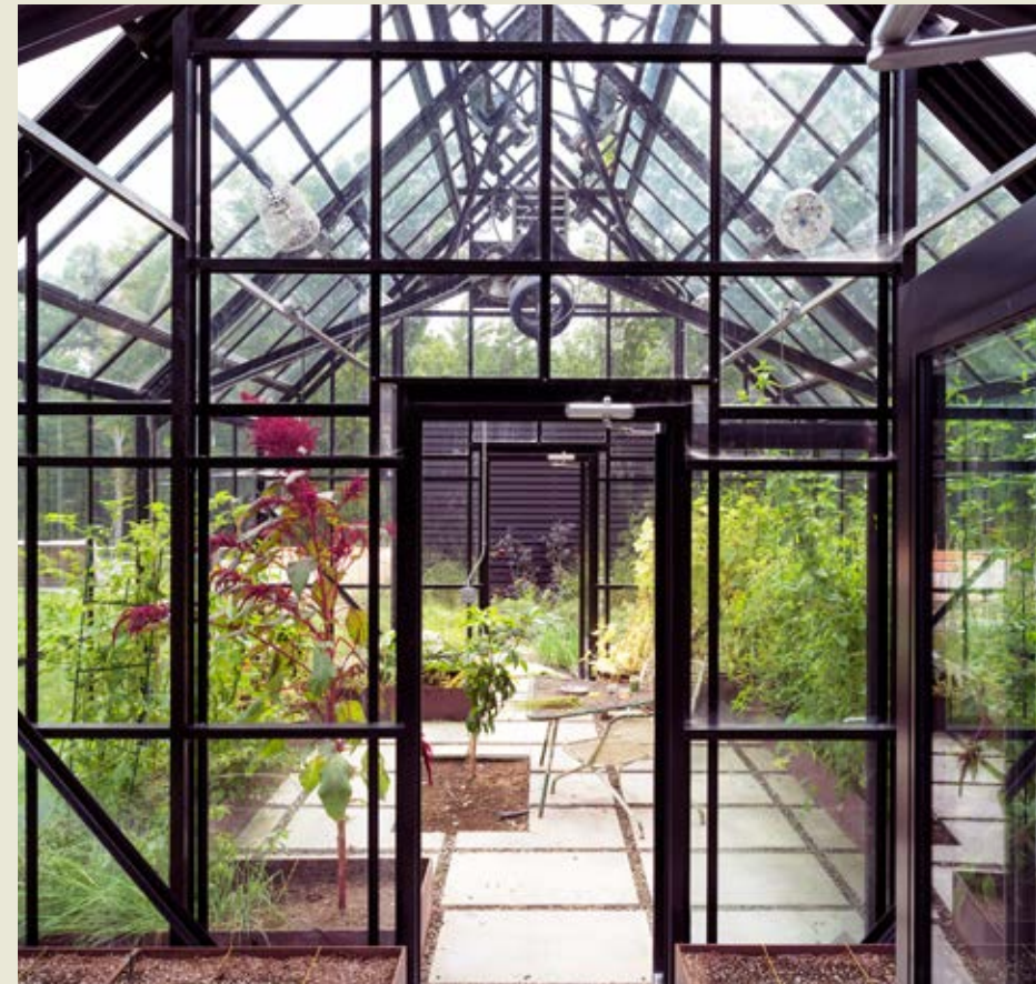
The partition wall in this greenhouse creates two distinct growing climates for optimum harvest.
